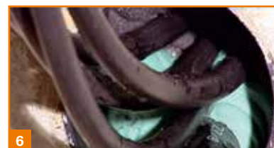
Lift the cables and apply STOPAQ® 2100 Aquastop with an appropriate application gun around the cables. Use the flexible nozzle to fill 100mm of the duct without air enclosures. Apply from the rear of the duct to the front.
