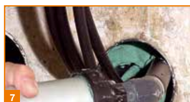
Apply STOPAQ® 2100 Aquastop up to 50mm from the front of the duct.
