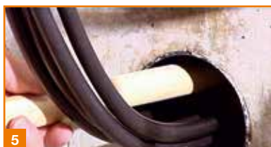
Make sure that the barrier is applied 150mm inside the duct.
